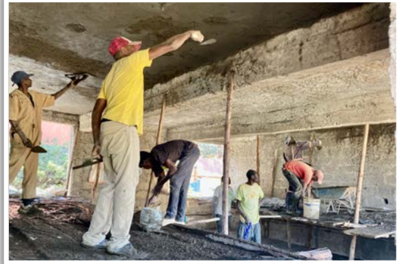
Workers are finishing the inside plaster of the classrooms.
